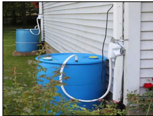
Hose connection from downspout diverter to barrel should be positioned without sags or loops to allow free flow of rainwater into the barrel. Downspout diverter should be placed 2 feet above the rain barrel. Credit: Chagrin River Watershed Partner, Inc.
