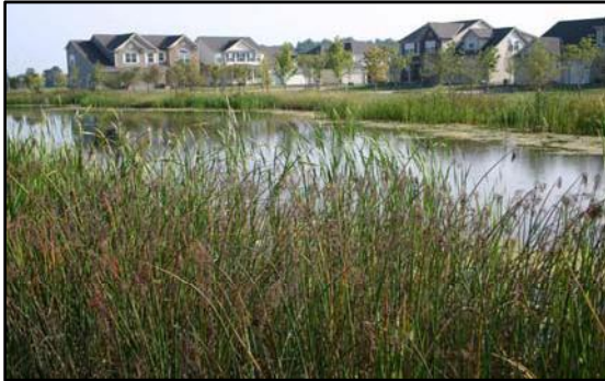
Wet pond with maintained shoreline containing aquatic bench for wetland vegetation to improve pollutant removal. Credit: Ohio Department of Natural Resources Division of Soil & Water Resources.
