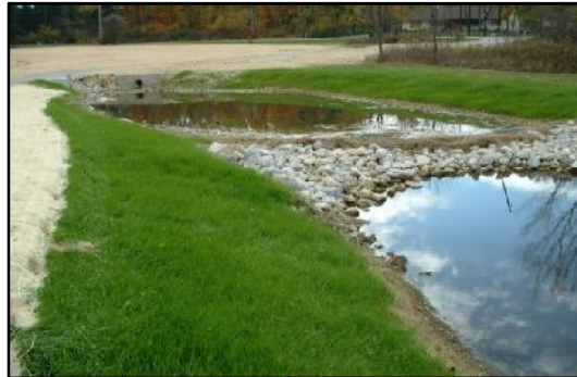
Wet pond containing a forebay pool to capture sediment entering the wet pond from the storm sewer inlet pipe visible in the background. Captured sediment is periodically removed from the forebay area. Credit: Summit Soil & Water Conservation District
