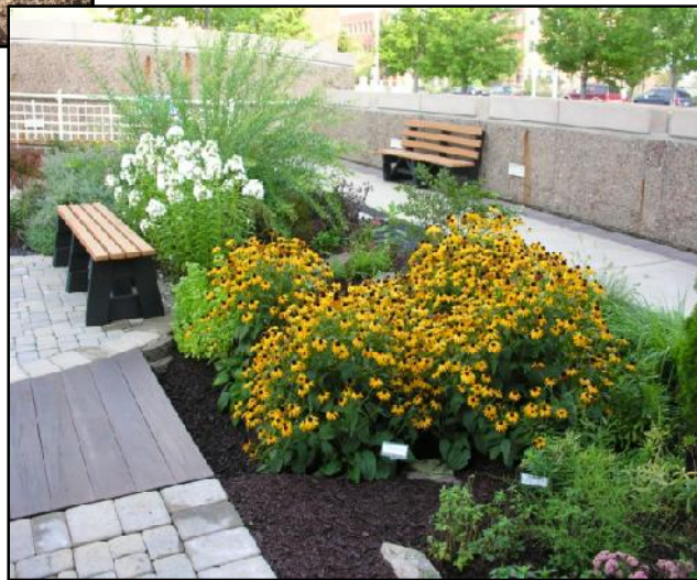
Fully mature rain garden capturing runoff from paved surfaces at the Northeast Ohio Regional Sewer District administrative offices in Cleveland. Credit: Northeast Ohio Regional Sewer District
